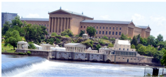
The old Fairmount Water Works sits below the Philadelphia Museum of Art
